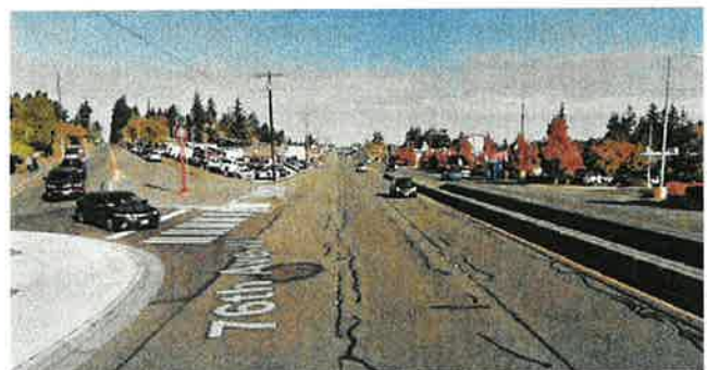
Type-C curbing and raised concrete barrier median at intersection of 76th Avenue and Highway 99 between 224th Street and 228th Street
